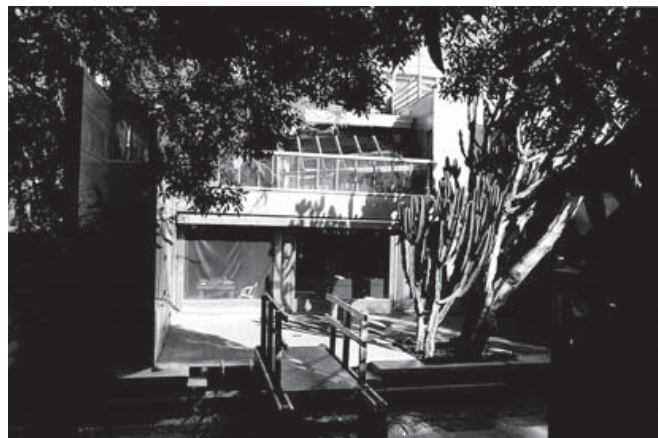
Figura 1. Gehry Residence (1978), Santa Monica, Los Angeles
